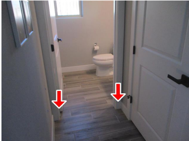
7.1 Item 3 (Picture) Bathroom hall
