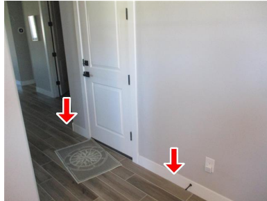
7.1 Item 4 (Picture) Garage hall
